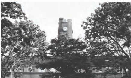
Research Center for Advanced Science and Technology (RCAST), The University of Tokyo
